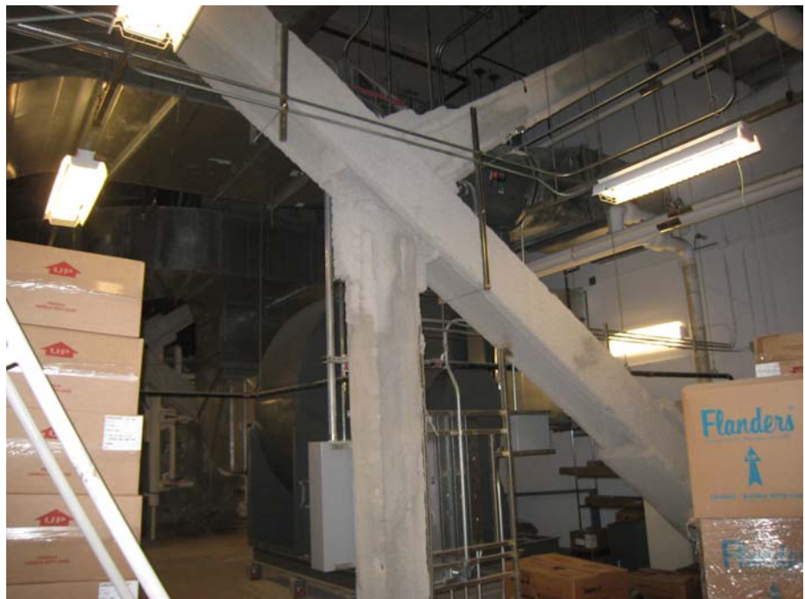
Figure 35: Outrigger on 28 th Floor
