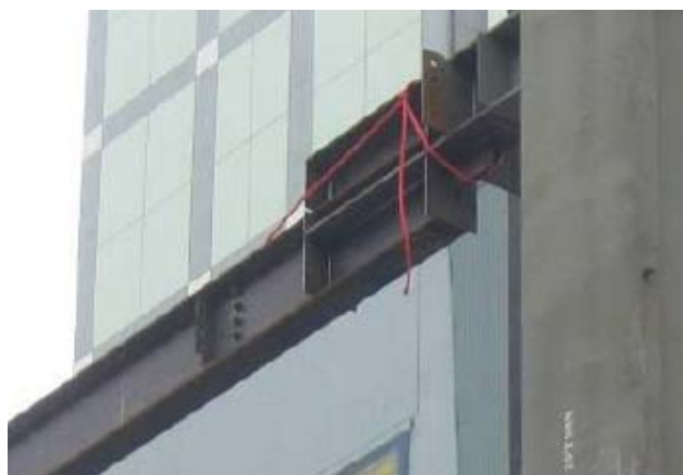
Figure 3: 'Dog-leg' beam connection, courtesy of Thornton Tomasetti
