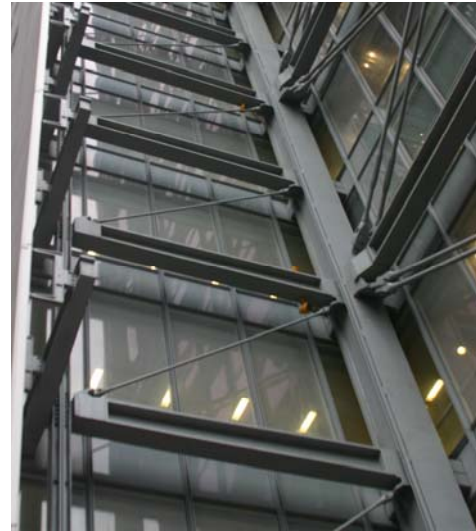
Figure 7: Cantilevered bays from exterior
