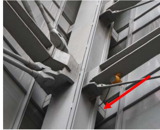
Figure 4: 'Dog-leg' penetrating building envelope
